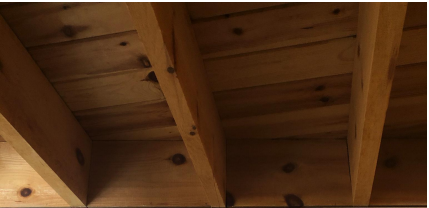
Exposed floor joists and structural decking may be used for the roof structure and finish. No painting or other finish is required, saving on labour and material costs, and providing a pleasant organic aesthetic.
