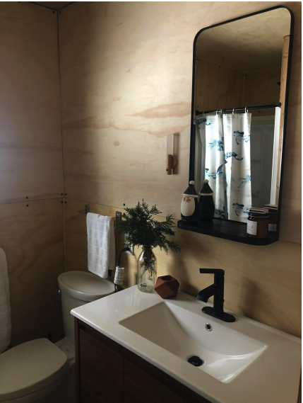
This bathroom is finished with a 1/2" G1S sanded Birch Plywood finish. The lower 4x8 sheet is treated with a water resistant coating (low VOC Varathane). No seam finish is required, simple black anodized button fasteners and inexpensive floor screws complete the look. This permits easy repairs and additions over the long term while concealing cavity spaces.
