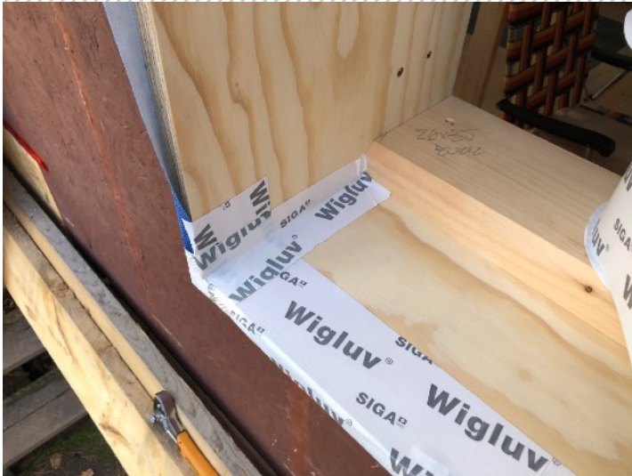
1-3. Just to give an idea of interior buck corner taping to guide any water away and out, lapping layers up and over the back dam
