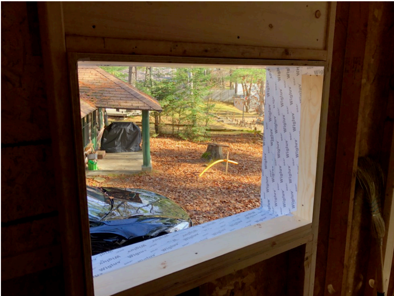
This is a redundant step, but it's good to have a waterproof sill at the very least, which is why we tape off the plywood buck sill right up and over the back dam. An additional layer of Majvest SA gets added to this.
