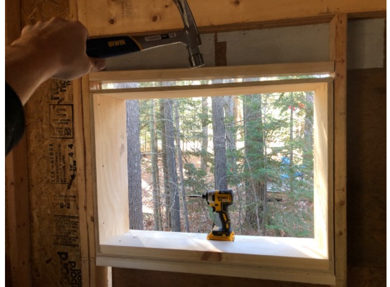
Where possible, structural framing can even frame tight to the window buck, making for fewer gaps to air seal. In this case, the window is in a renovated wall so we could frame below an existing header and support the buck with a simple 2x4 frame around the plywood buck. Note the impact driver is sitting on the sill below the back dam.
