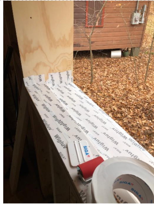
1-3. Just to give an idea of interior buck corner taping to guide any water away and out, lapping layers up and over the back dam
